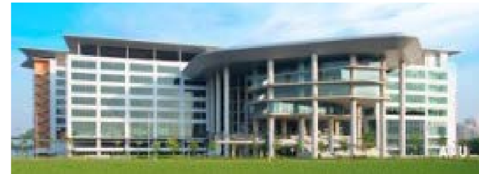
APU's purpose-built campus with an ultra-modern design is strategically located at MRANTI Park Malaysia in Kuala Lumpur.
