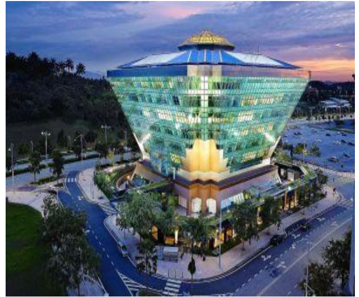
Fig 3 The Energy Commission's Diamond Building Putrajaya
