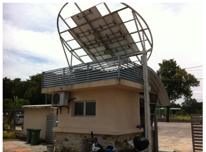
Guard House Operating on Self Generated Power
