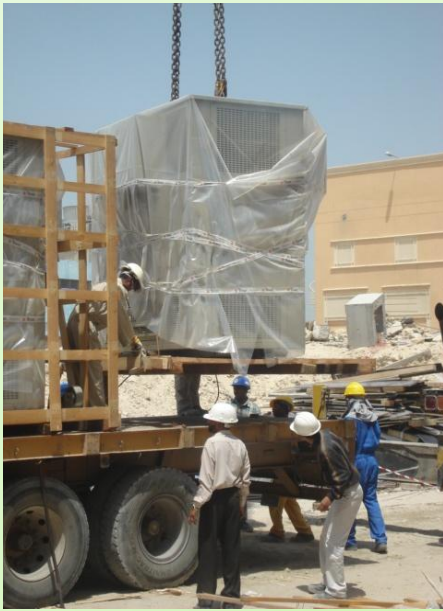
Heavy Equipment Offloading at A Construction Site – DCP 1, Gardens Project
